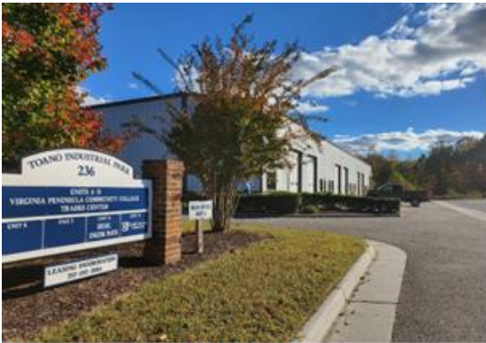
Pic 1: Toano Site - Steel Frame Building
