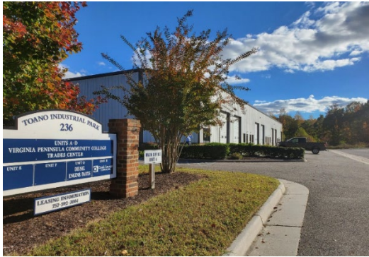
Pic 1: Toano Site - Steel Frame Building
